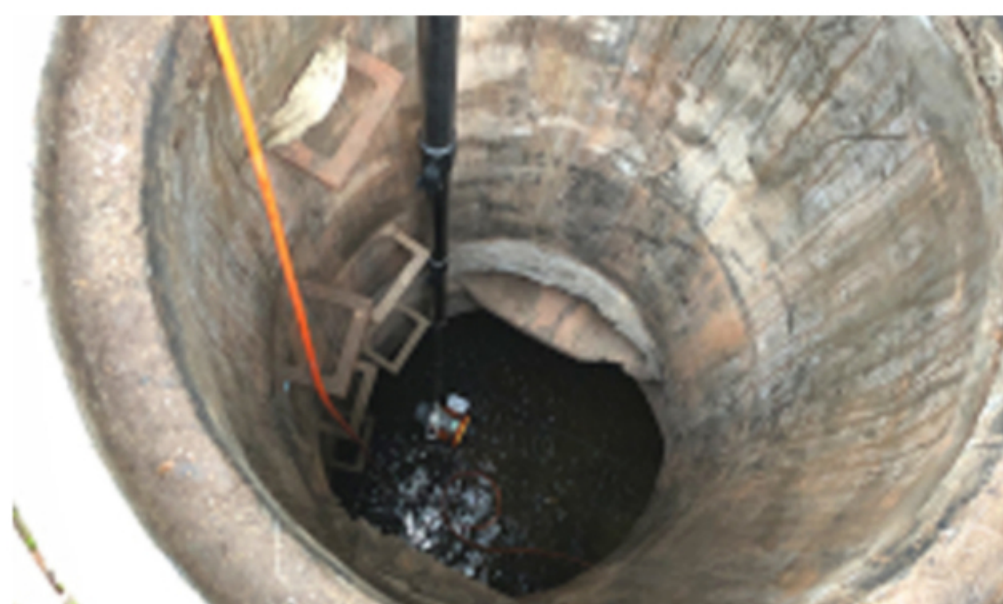
Municipal rainwater and sewage pipeline inspection
