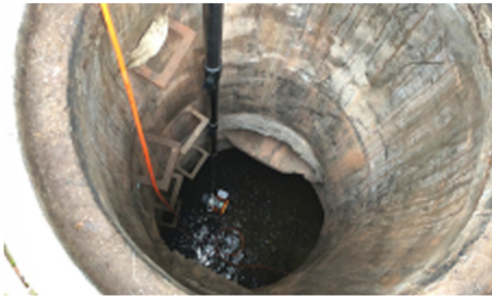
Municipal rainwater and sewage pipeline inspection
