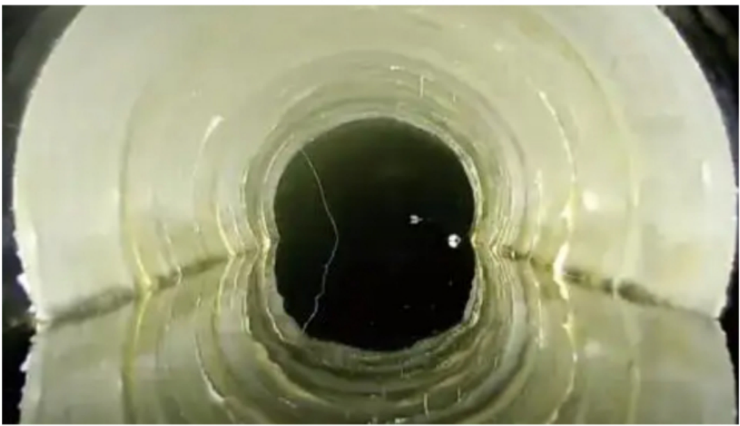
Pipeline repair construction observation
